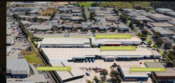
WETHERILL PARK NSW
